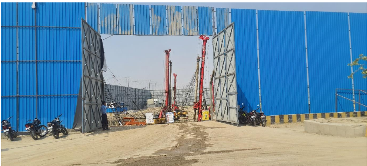
Figure 8 Site Barricading
