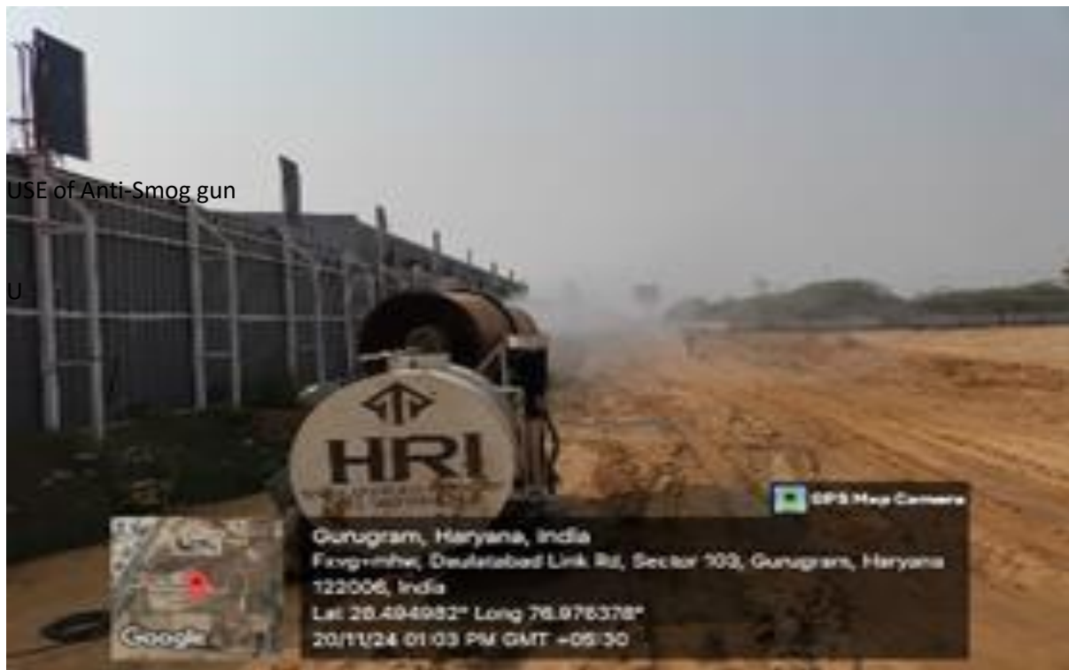
Use of Anti-Smog gun at site
